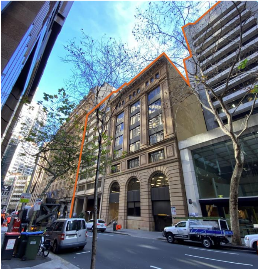
Figure 4: View from O'Connell Street, including the former Rofe Chambers heritage item at No. 19 O'Connell Street
